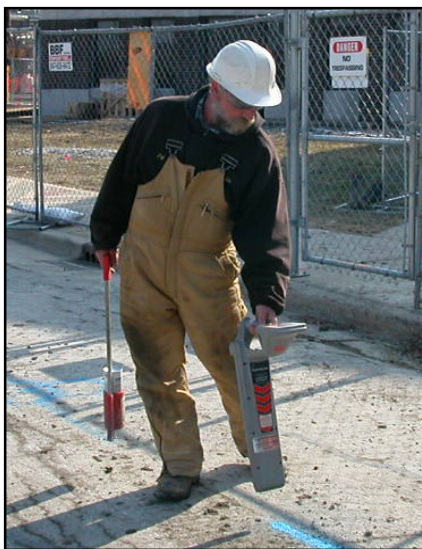
"Critical Dig" Location Specialists
