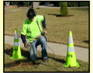
Step 1. Leak Detection
