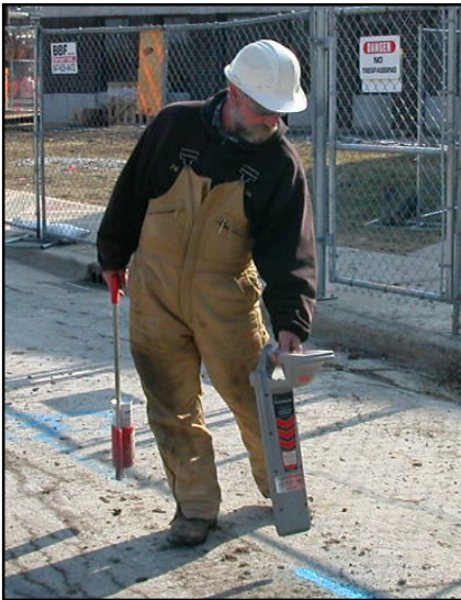
"Critical Dig" Location Specialists
